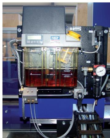
Fig. 19: Oil Air Lubrication
